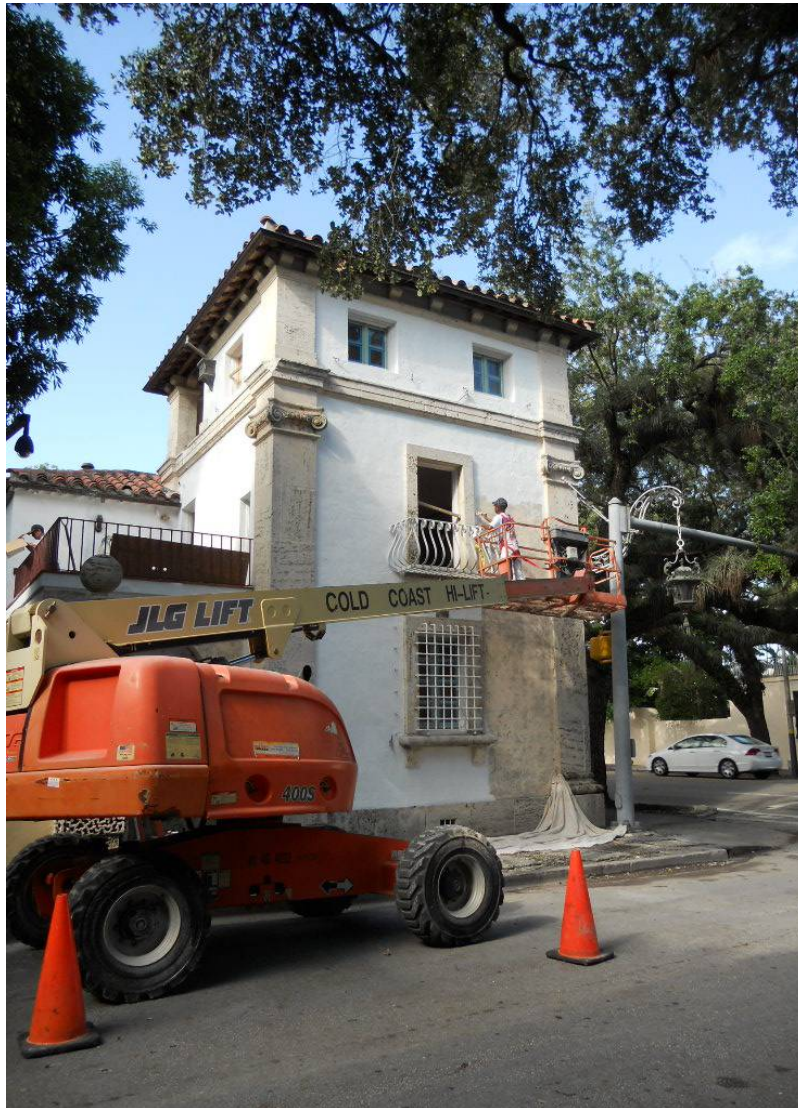
Painters add finishing touches to the East Gate Lodge renovation.
