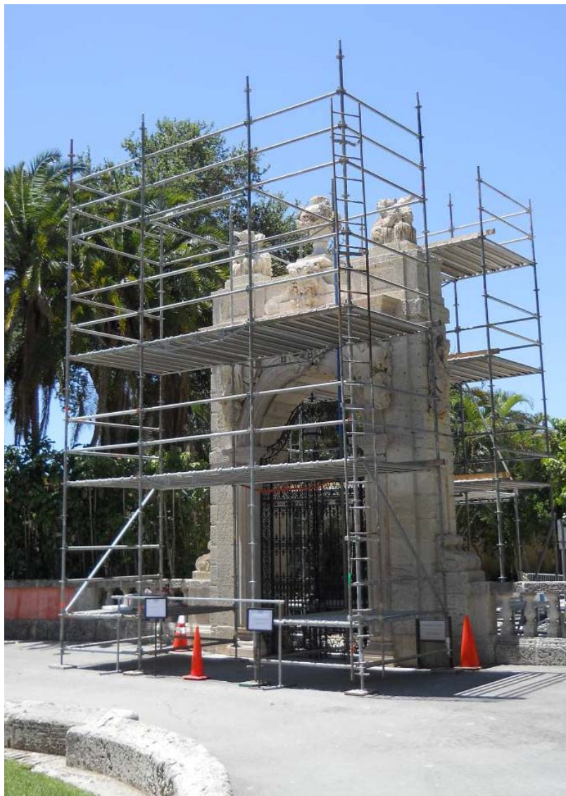
One of the two Forecourt Gates under conservation treatment.
